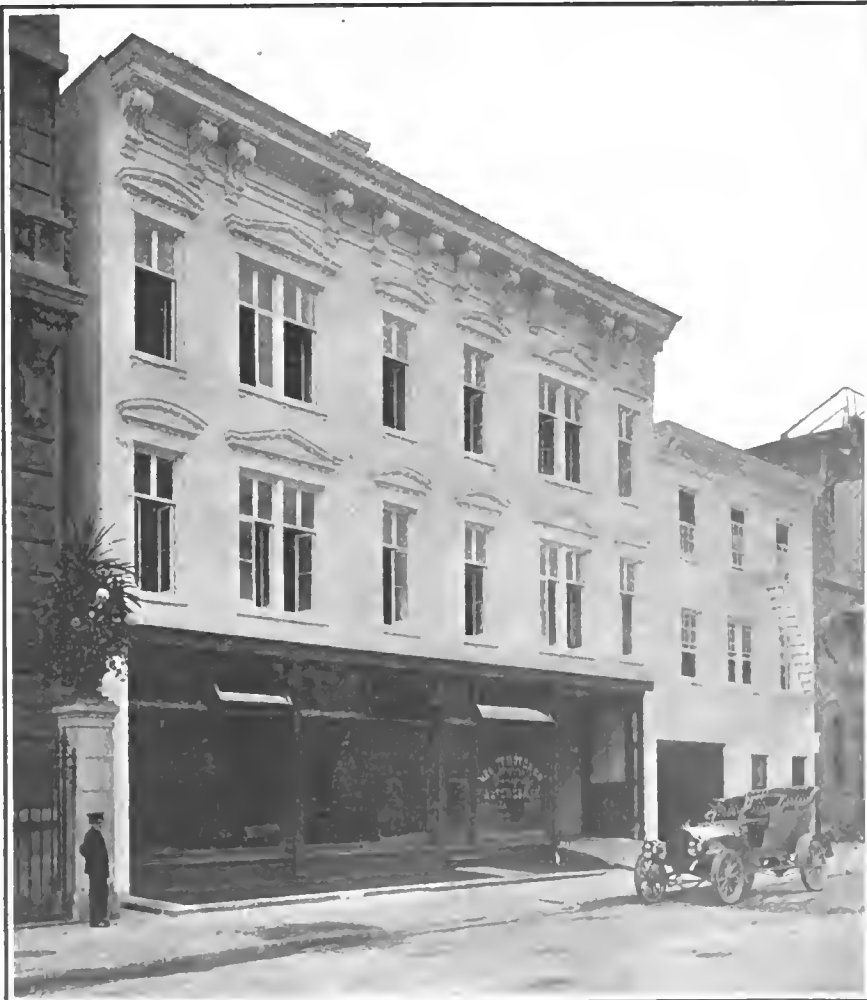
HEWITT MOTOR COMPANY'S GARAGE ON EAST THIRTY-FIRST STREET, NEW YORK.
